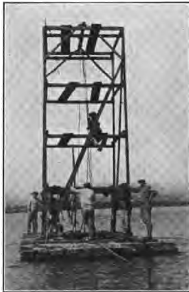
FIG. 7.—A boring rig for river and harbor work.
